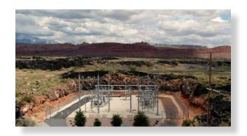
The Paul Grimshaw Substation is our newest Substation. It contains two 10 MVA transformers that convert the transmission voltage from 69,000 volts to 7,200 volts to be delivered on the distribution circuits. There are six distribution circuits coming out of this substation.
