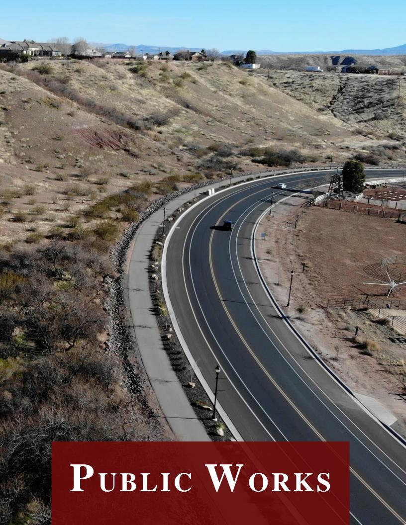
The Public Works department is responsible for maintaining 48 miles of roadway, curb, gutter, and sidewalks throughout the City. This includes asphalt placement and preservation, traffic control, street signs, striping, chip-seals, crack seal, slurry seals, traffic signals, street sweeping, and sidewalk repairs. The Fiscal Year 2023 budget is \$1,059,765 which is a decrease of 17% from FY 2022.
