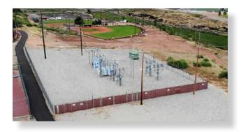
The Parley Hassell Substation contains one 10 MVA transformer and has 4 distribution circuits coming out of it. This is our oldest substation and we are in the process of upgrading it with new controls.
