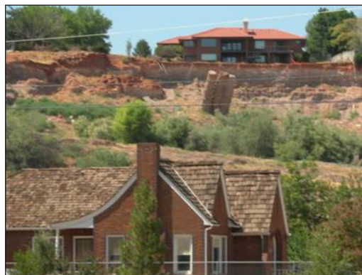
Figure 1-7: Hillside failure due to hazardous soil conditions.
